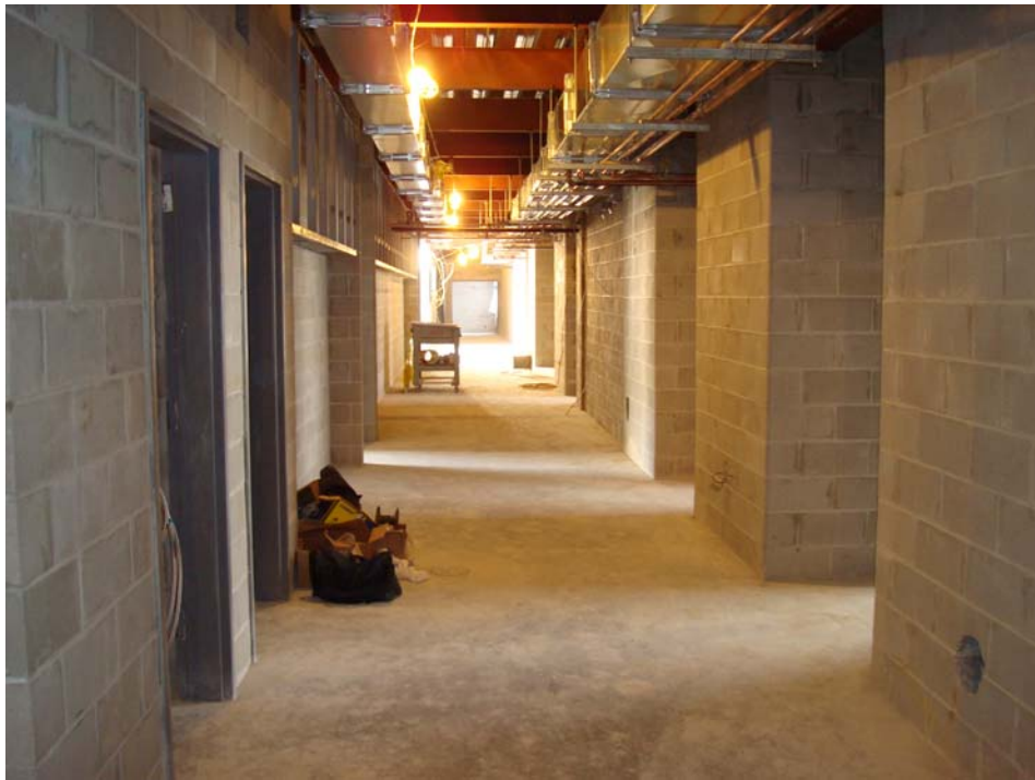
Second Floor Corridor.
