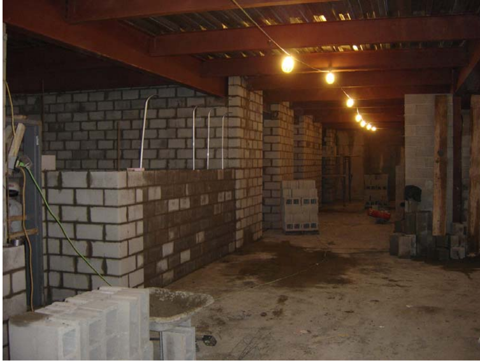
Progress of interior CMU walls.
