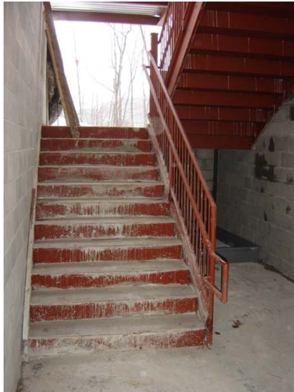
Stair installation (poured concrete steps).
