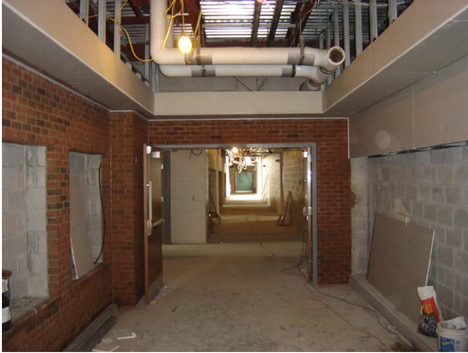
Sheetrock installation at soffits.
