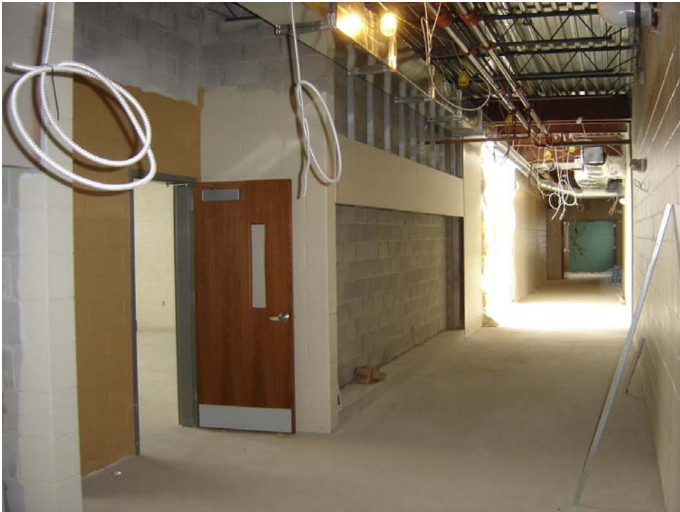
Wood door installation at third floor classrooms.
